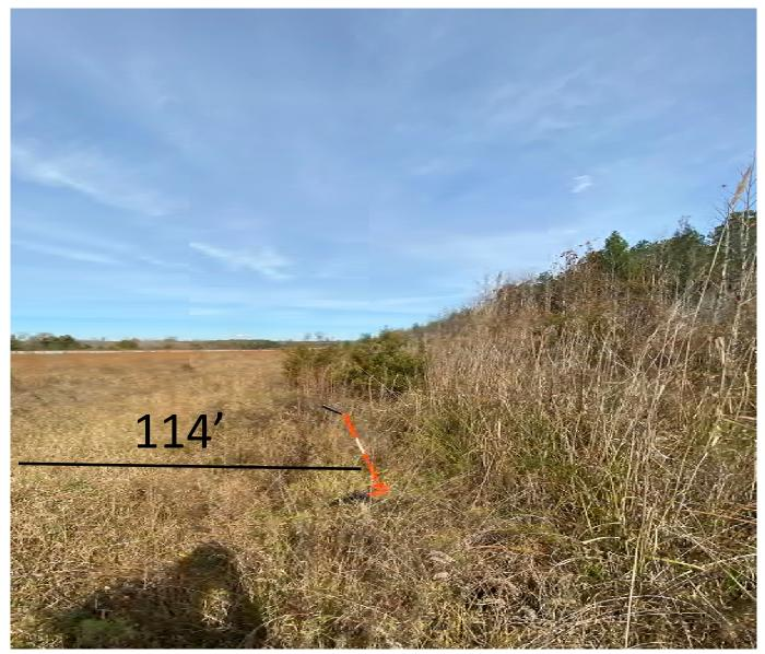
Violation: Primary Surface <u>DOES NOT MEET</u> state licensing standards. Ensure grass and trees are cut and removed from of the Primary Surface. 114' to runway centerline; 125' from centerline is required.
