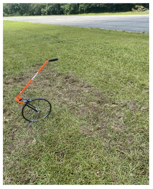
**VIOLATION** Runway Safety Area **Does Not Meet** state licensing standards. There are ruts located in the Runway Safety Area. Please repair ruts and ensure that the ground is level and smooth.
