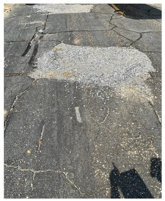
Apron surface is **<u>POOR</u>** in condition. Extensive longitudinal and transverse cracking, with complete failures in certain places.
