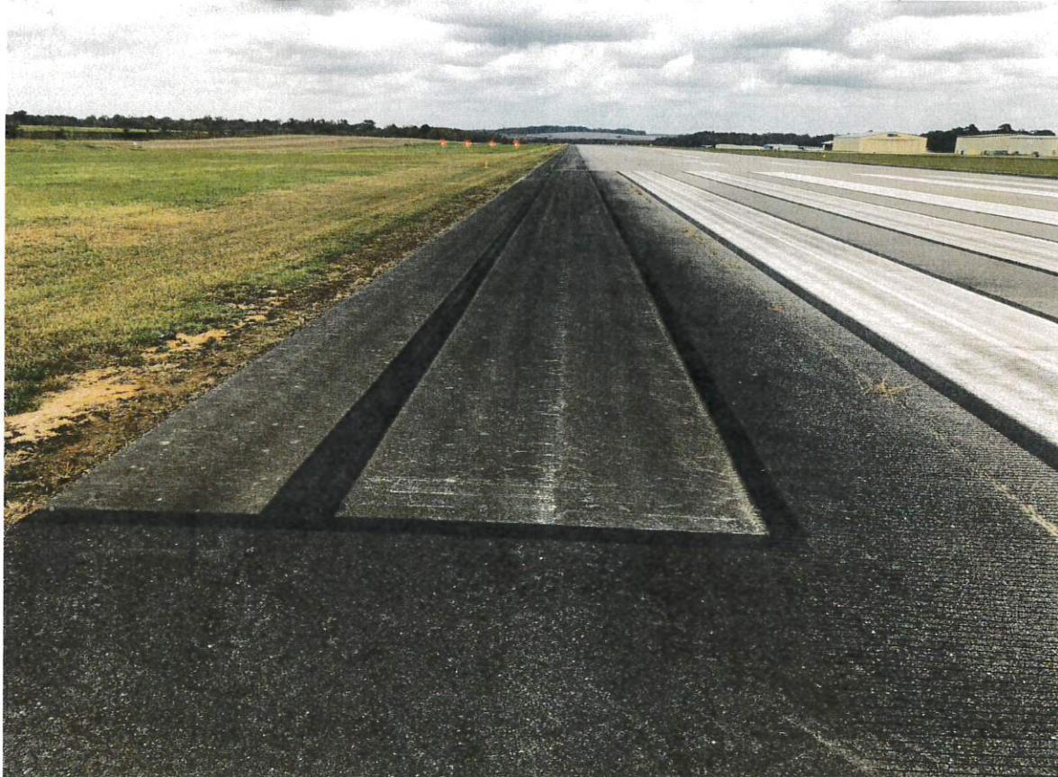
Photo # 5 – PIR Markings Runway 36 (Edge Obscuration)
