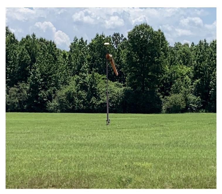
Wind direction indicator is in <u>POOR</u> condition and should be replaced.
