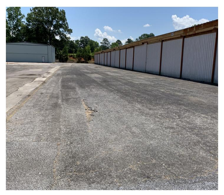
The old taxilanes are in <u>POOR</u> condition, exhibiting extensive cracking and raveling, which is producing foreign object debris (FOD).
