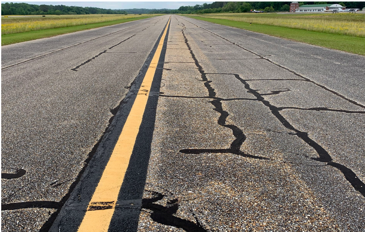
Photo #7— Crack Seals
