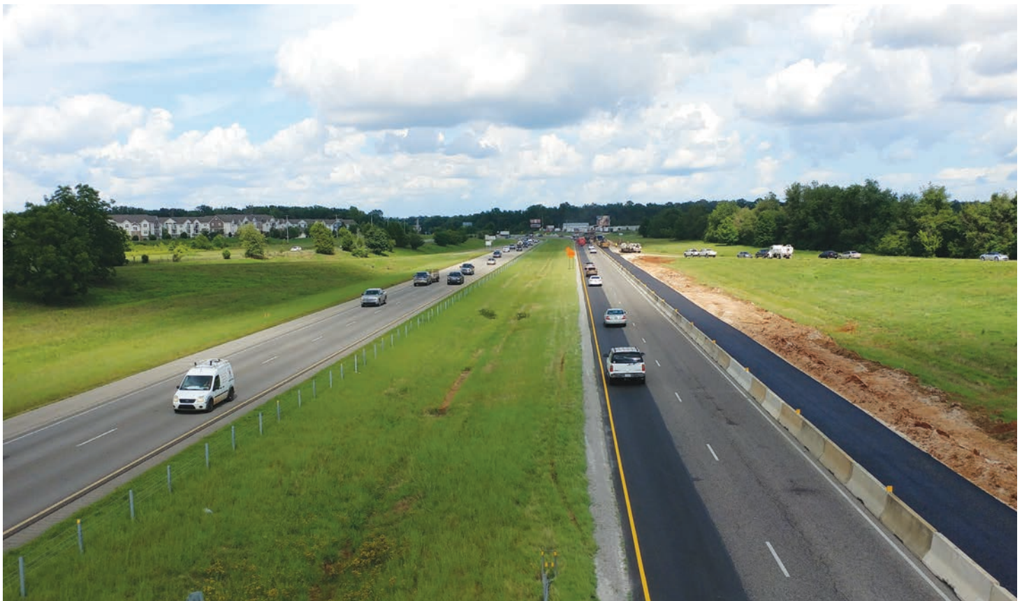
Pictured above is part of the I-565 expansion project.
