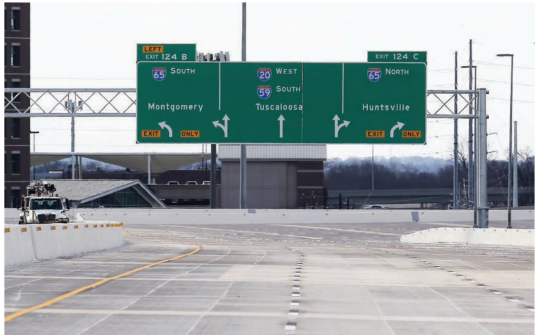
A new portion of the I-59/20 bridges heading westbound.
