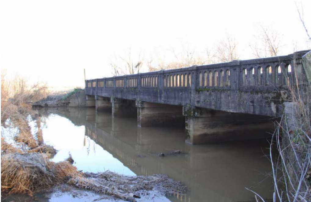
Side View BIN 000558 (Photos courtesy of Garver)
