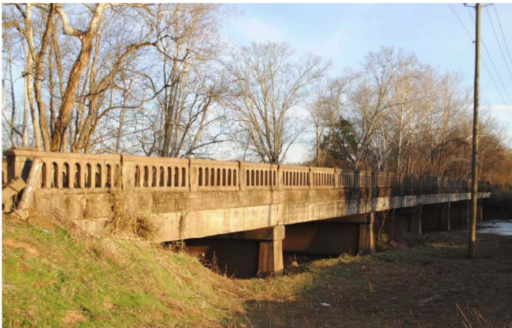
Side View BIN 000559 (Photos courtesy of Garver)
